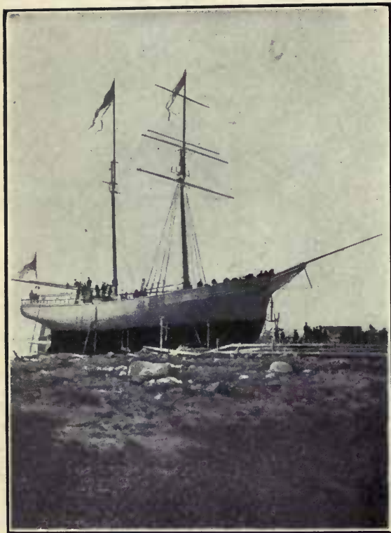
TYPICAL TOPSAIL SCHOONER AND LAUNCHING. Barrington Rig, built at Warren Doane's Yard.
